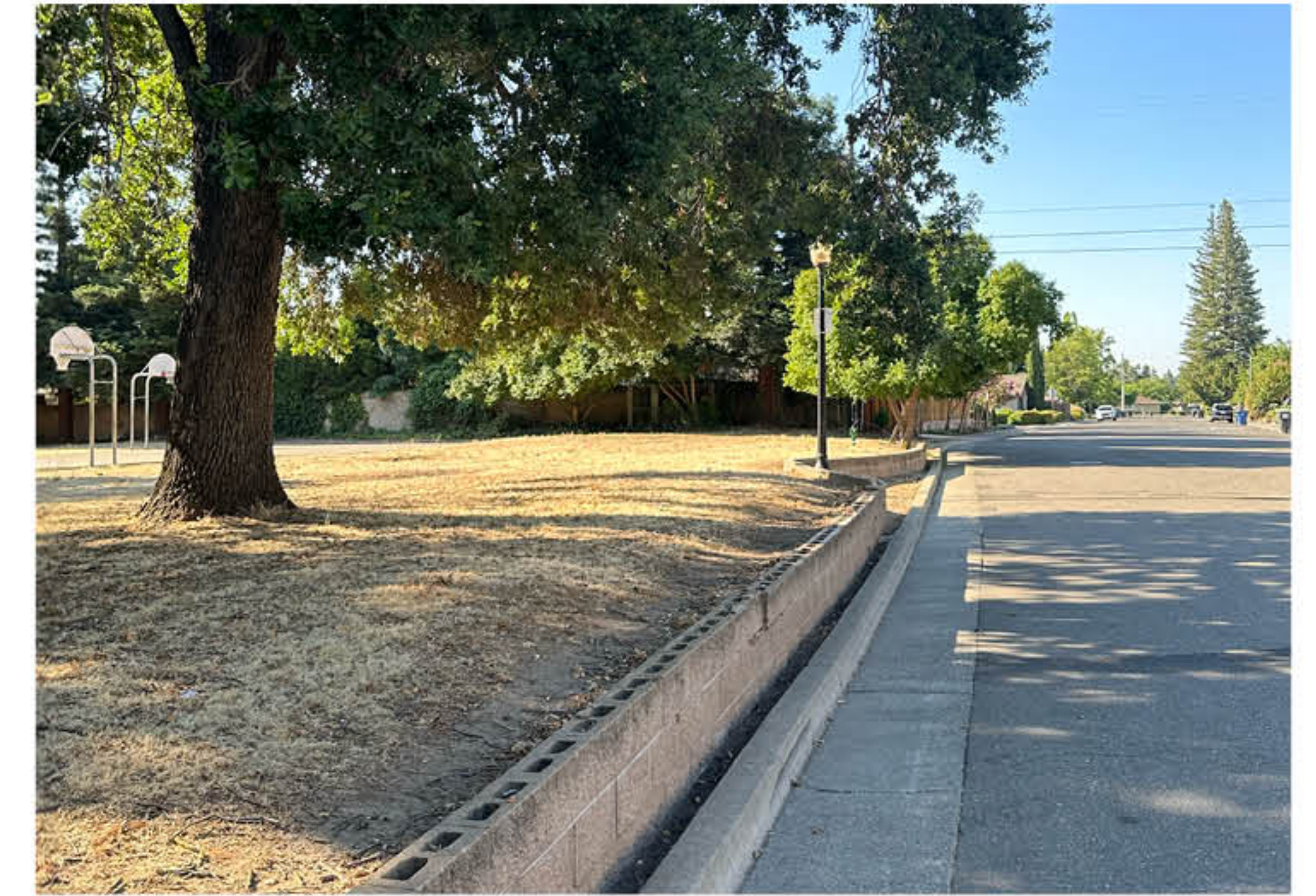
View of Retaining wall along Glancy Dr. looking South
