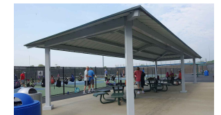
SHADED PATIO NEXT TO PICKLEBALL COURTS
